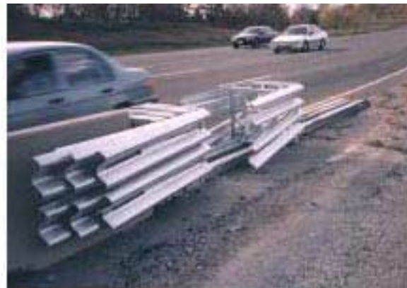
Damaged TRACC Prior to Replacement
