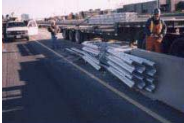
TRACC Replacement in Progress
